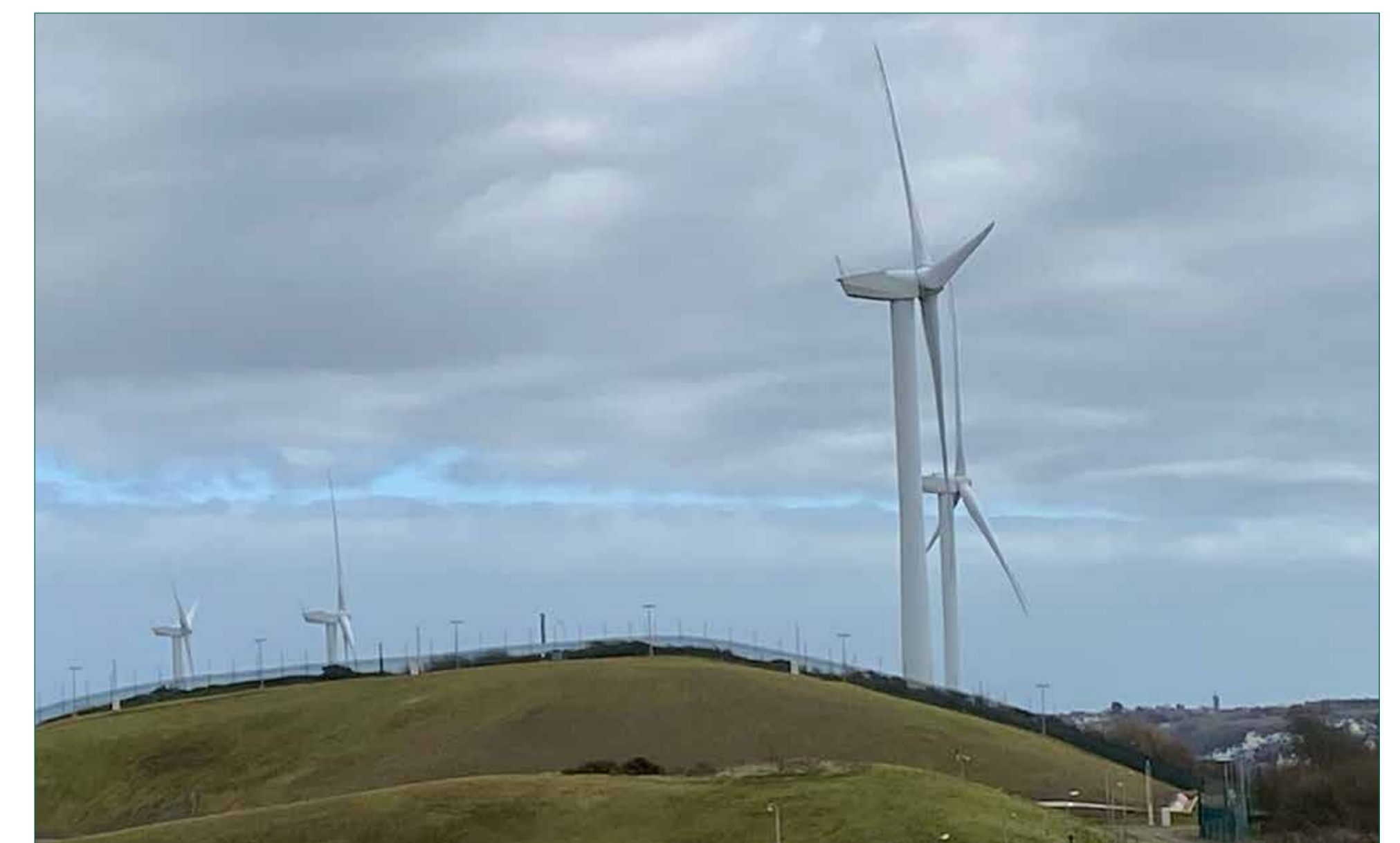
EXISTING WEAR POINT TURBINES WITH SOLAR FARM
