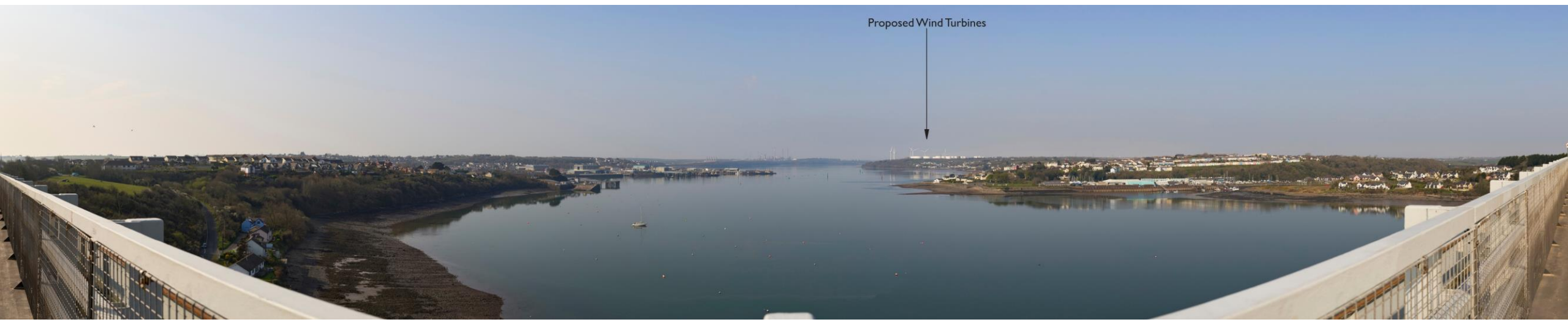
Photograph C: View from Cleddau Bridge
